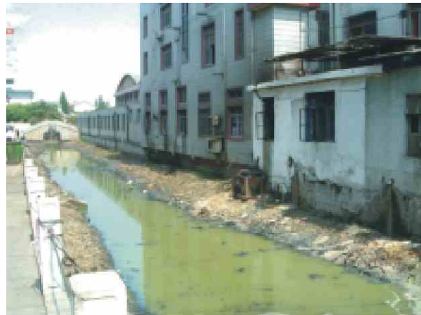
HuaXin / Shanghai / China; May 2003: The wastewater situation required an ecological and economical solution. The demand of the local government was to reach this result the local facts should be used.
