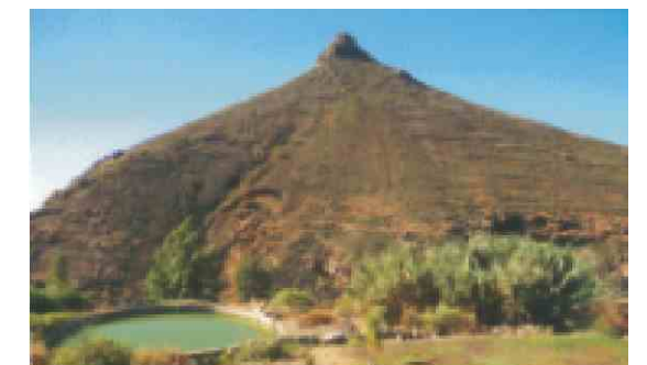
Constructed wetland purifying the wastewater of a restaurant. The outlet is collected in a big basin for garden irrigation. El Refugio, Tenerife, Spain
