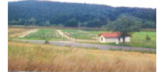
This plant is suitable for the wastewater of 400 inhabitants including stormwater overflows Odenachsen, Germany
